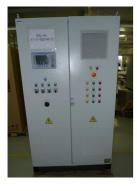
Basic and detail design of automation, DC drives, cables, field instrumentation and connectors for DC driven drilling rig. Manufacturing and delivery of all cabinets for control system, DC drives for mud pumps, drawwork, and rotary table for truck mounted mobile drilling rig BU 2500. Delivery of signal and power (high current) connectors. Total installed power in DC drives is 1,9 MW. Used PLC control system Allen-Bradley CompactLogix,
