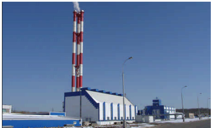
MosTeploEnergó's Lublino heating station in Moscow.
