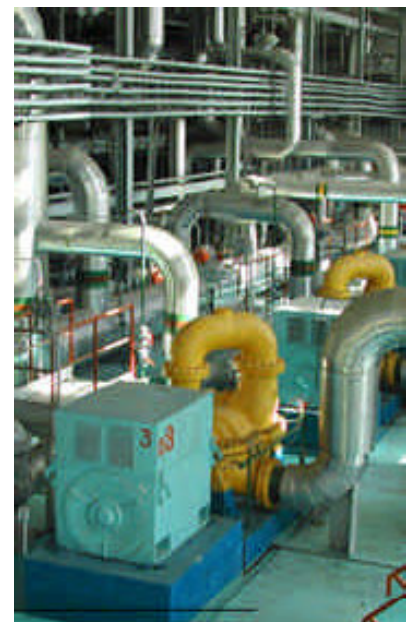
Main pumps and motors at Lublino heating station.
