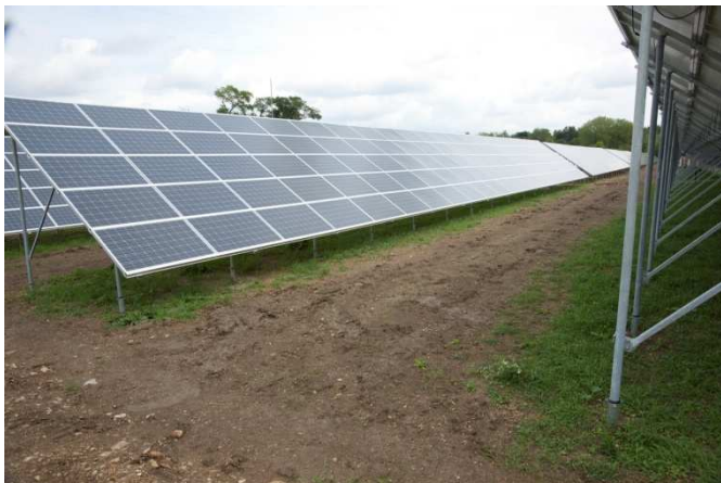
Figure: Photovoltaic modules organized into rows
