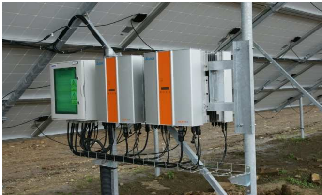
Figure: AC/DC cabinet and solar inverters Delta Solivia 5.0 located below photovoltaic modules
