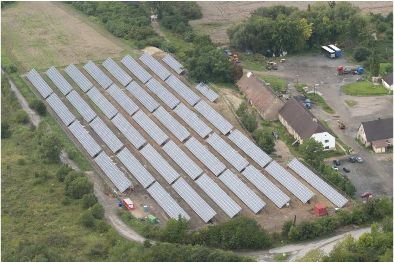
Figure: General view of photovoltaic power plant. Photovoltaic modules are arranged into groups, transformer kiosk in right bottom corner.
