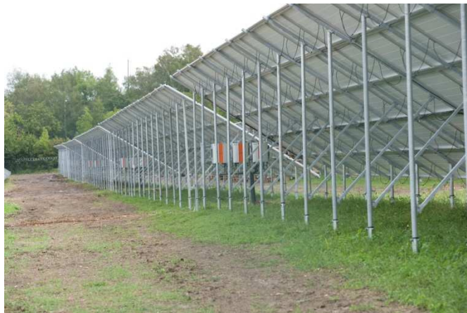
Figure: Solar Inverters Solivia 5.0 below PV modules
