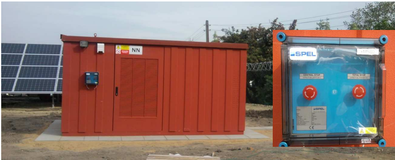
Figure: 1MW transformer kiosk, safety pushbuttons (in front)
