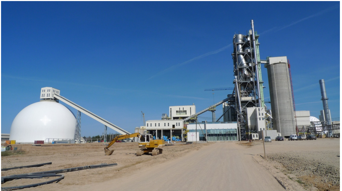
Figure: Main view to cement plant: Pre-heater and raw silo (on right), Main bag house, Central Control Room and clinker cooler area (middle), clinker storage (on left),
