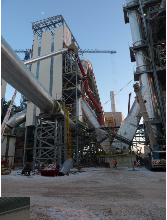
Figure: Pre-heater: Pre-heater tower (four stages) and view to rotary kiln (left figure); Pre-heater ID fan, 3,8MW (right figure) and MV VFD for ID fan ( figure bellow).
