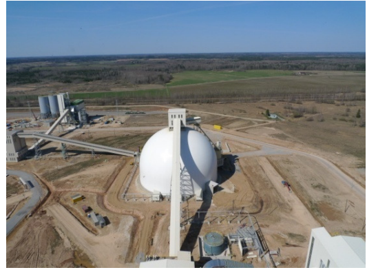
Figure: Clay and limestone storage. Clay dryer area (in front). Figure on right: clinker storage, cement (final) mill and expedition area (on back)
