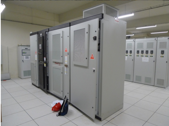
Figure: Clinker cooler: MV VFD for ID fan, air cooled, 1000kW, 6,3kV; technology –clinker cooler (underlying)
