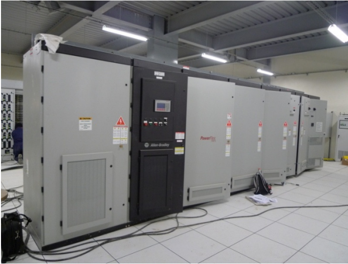
Figure: Raw mill: MV VFD for ID fan, liquid cooled, 4,5MW, 6,3kV; input/output and bypass section cabinets (figure on right)
