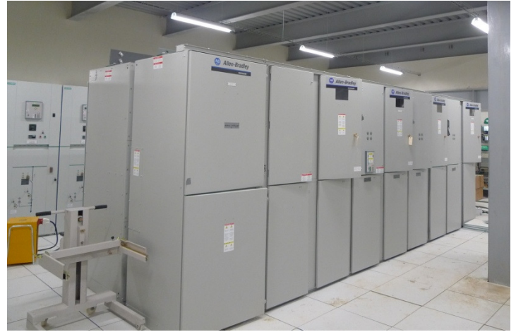
Figure: Raw mill: MV VFD for ID fan, liquid cooled, 4,5MW, 6,3kV; input/output and bypass section cabinets (figure on right)
