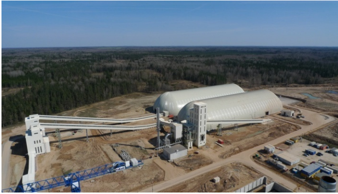
Figure: Clay and limestone storage. Clay dryer area (in front). Figure on right: clinker storage, cement (final) mill and expedition area (on back)
