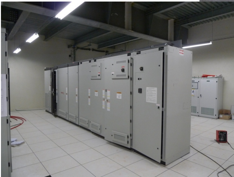
Figure: Pre-heater: Pre-heater tower (four stages) and view to rotary kiln (left figure); Pre-heater ID fan, 3,8MW (right figure) and MV VFD for ID fan ( figure bellow).
