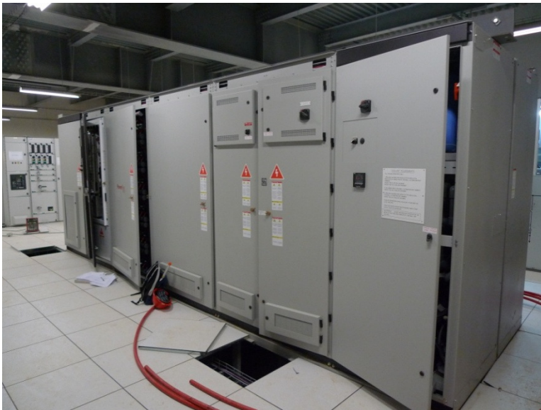
Figure: Raw mill: MV VFD for ID fan, liquid cooled, 4,5MW, 6,3kV; input/output and bypass section cabinets (figure on right)
